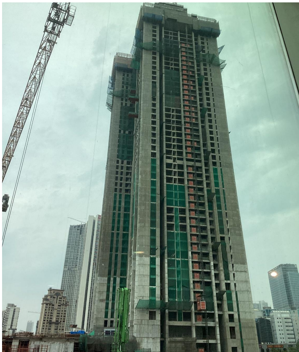
Exhibit 41: Birla Niyaara – Phase 1 construction on schedule; 53 floors constructed
