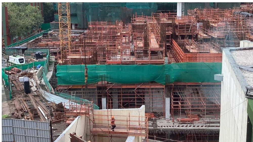
Exhibit 42: Birla Niyaara's P-2 – Basement construction complete; execution progressing well
