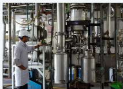
Multipurpose Pilot Plant
