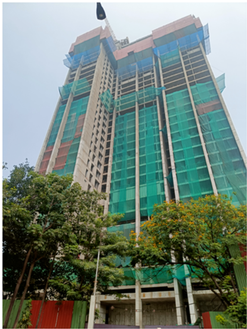
Fig. 3: ABRE: Niyaara Tower under construction
