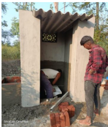
Toilet construction in Siludi
