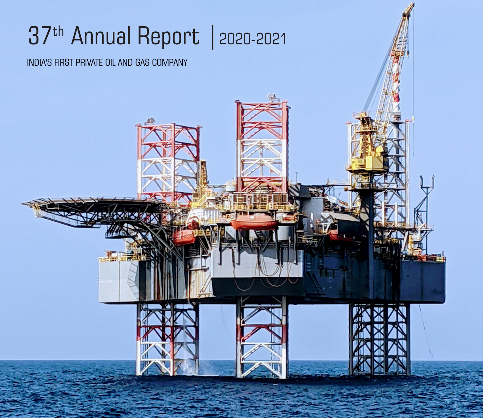
Offshore Installation at B-80
