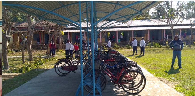
Cycle shed constructed at Powai School
